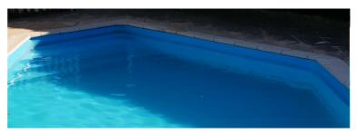
The image above right is of a liner that is only around three years old, but has permanent stains at the water line. There are two reasons for this – poor or irregular maintenance, and excessive use of sun-screen by swimmers – especially P20 cream. Whilst the liner isn't harmed by this, it's unsightly.
