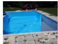
Most pools have a concrete floor, and this needs to be covered with a felt 'underlay' which must be glued into position. If the pool has concrete walls as well, then the felt needs to extend up the sides. It's essential that the pool is kept clean and free from any bits that will protrude and show as lumps under the liner. That's one reason why a windless day is needed – also, the felt is very light, so controlling it in a gale is not recommended if you value your sanity.
